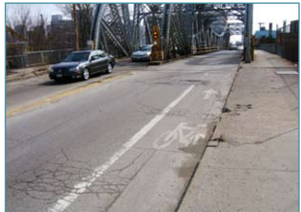
Halsted Street looking south at the river bridge
