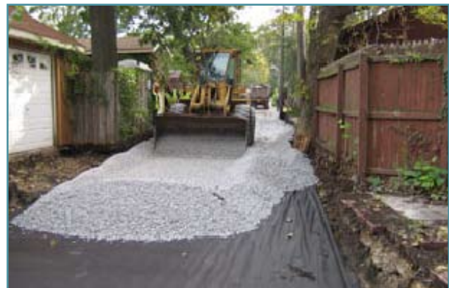
Permeable pavement being poured in an alley on fabric liner
