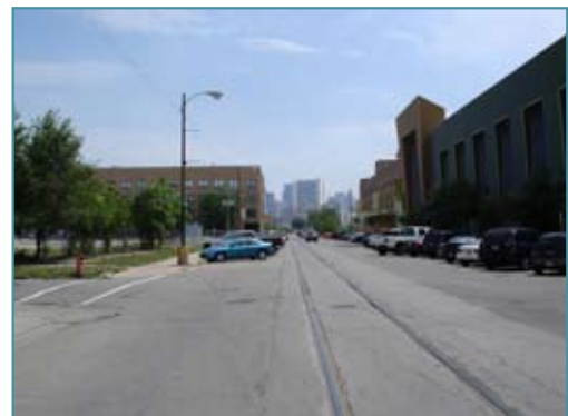
Various locations on Kingsbury Street showing parking on street and off street and the rails which are to be removed.
